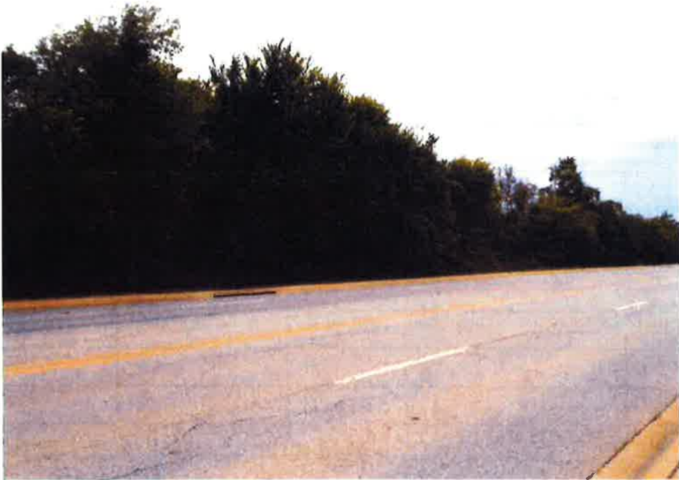
Whole Property Looking Northwest 7/27/2017
