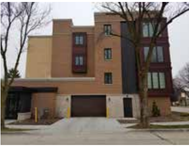
Parking within a building footprint. Parking contained at or half a level below grade within the walls of the building support three levels of apartments above with minimal surface parking. (Wauwatosa, WI)
