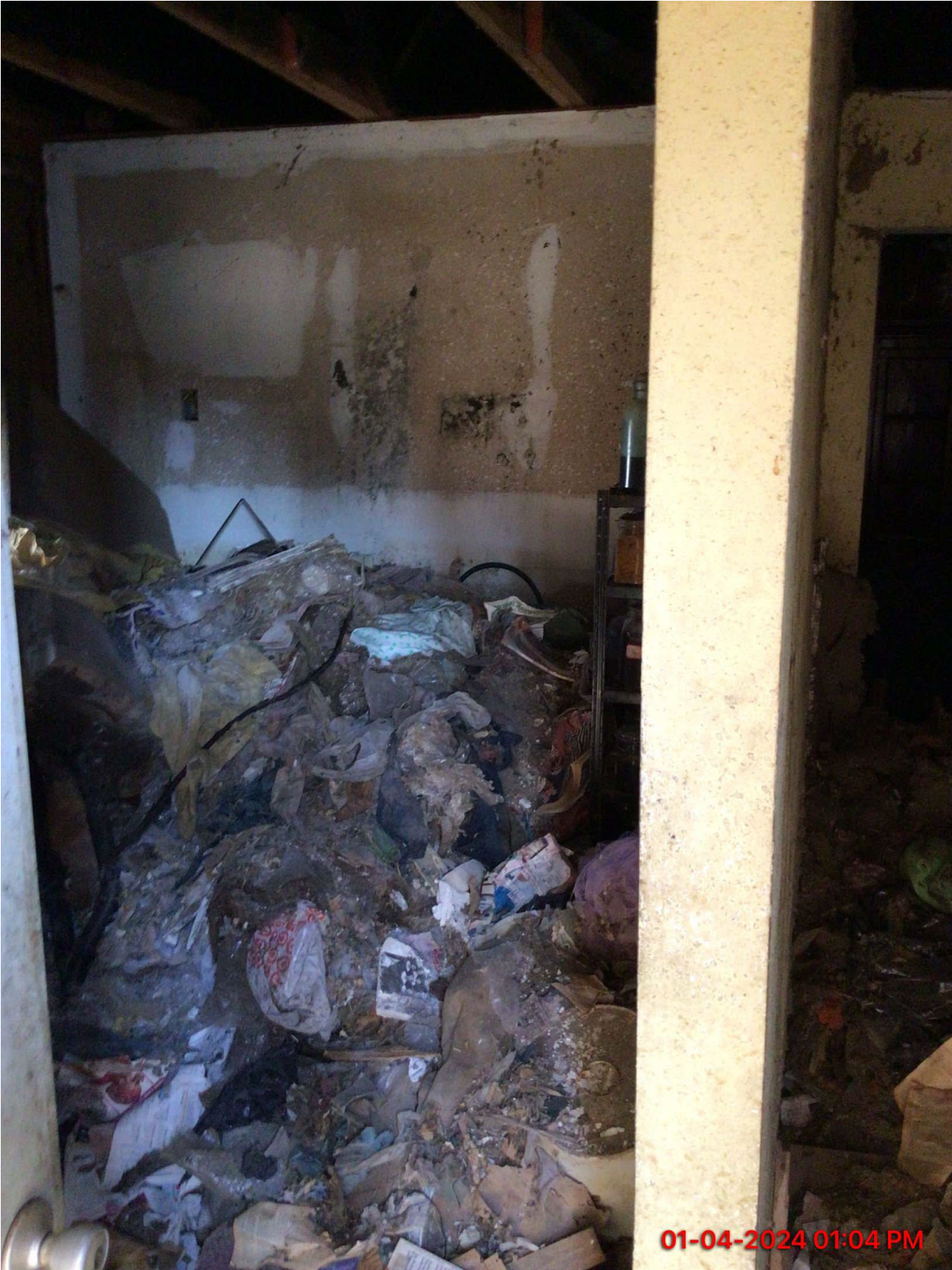
Inside the structure.
