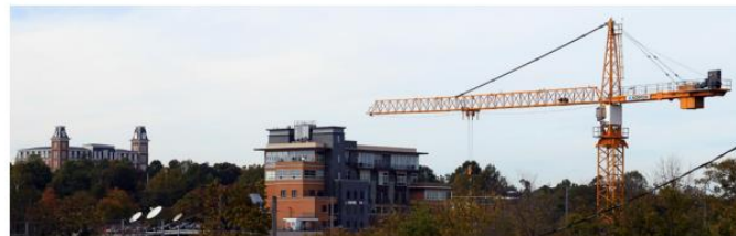
Photo 3.8 - Construction in Downtown Fayetteville
