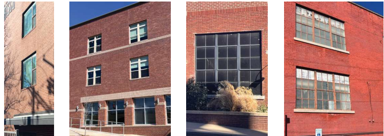
WINDOWS NON-OPERABLE THROUGHOUT* STANDARD GLAZING ON UPPER FLOORS ENLARGED GLAZING ON LOWER / PUBLIC LEVELS HISTORICAL WAREHOUSE SCALE AND PATTERN] *VARIANCE WILL BE REQUIRED AT TIME OF DEVELOPMENT
