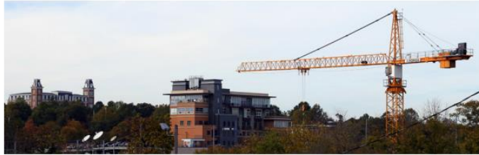
Photo 3.8 - Construction in Downtown Fayetteville
