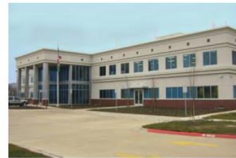
Photo 12.31 - Clean Technology Building
